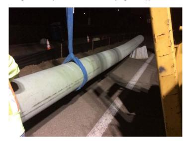
Figure 19: Pipe with Field Bend Laying on Supports
