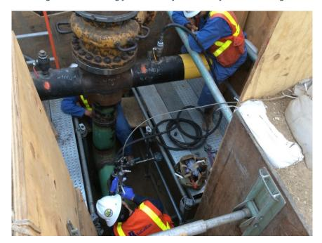
Any customers who were being fed by Compressed Natural Gas (CNG) or Liquified Natural Gas (LNG) have their service switched to being fed from the new pipeline. The process for abandonment of the original line also needs to take place. It begins by purging, isolating ends and taps, and permanently decommissioning the line which typically takes a few days to complete.
