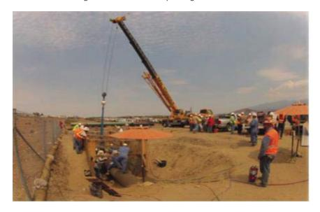
Figure 28: Checking for Leaks Before Start of Line Odorizing
