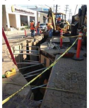
Figure 9: Shoring Installed in Pipeline Trench
