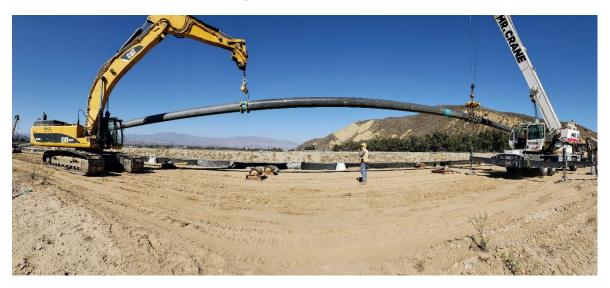
Figure 15: HDD Pullback
