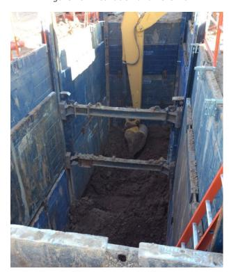
Figure 16: Excavation and Bore Pit
