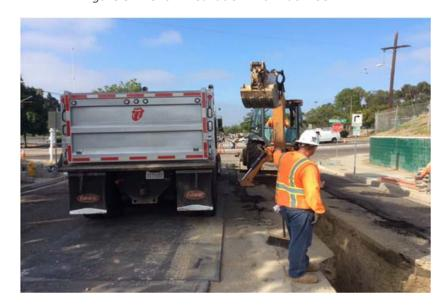
Figure 8: Trench Excavation with Backhoe
