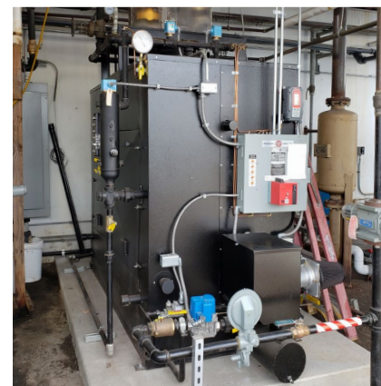
Hot water is essential for industrial laundry. When Pacific Uniform needed a new boiler, it chose a Parker Steam Boiler.
